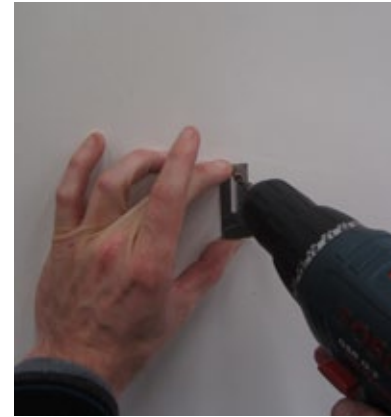
Place screw to fix staple. Colocar tornillo y grapa
